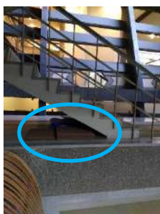
Under the stairs in front of Room C2
